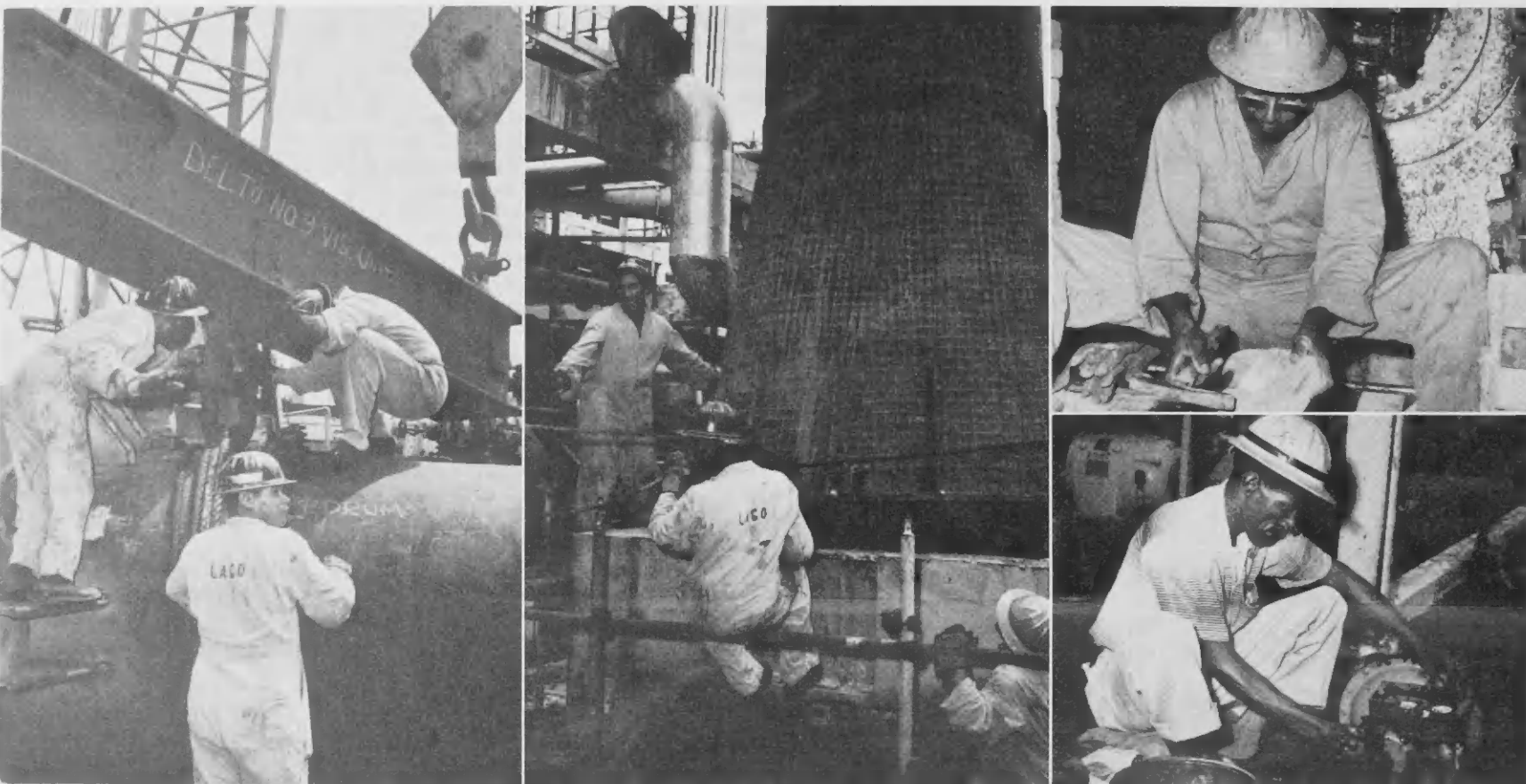
THE TURNAROUND features both big and little jobs. A derrick is used to position one of the base supports for a reaction chamber, left. The flared chamber base, center, is positioned on its new foundation. Chipping and cleaning, right, are important, too.
